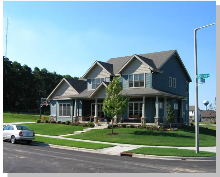
New housing should be characterized by designs that emphasize the architecture of the main body of the house, not the garage.
