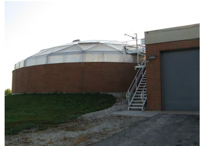
Biosolids storage tank
