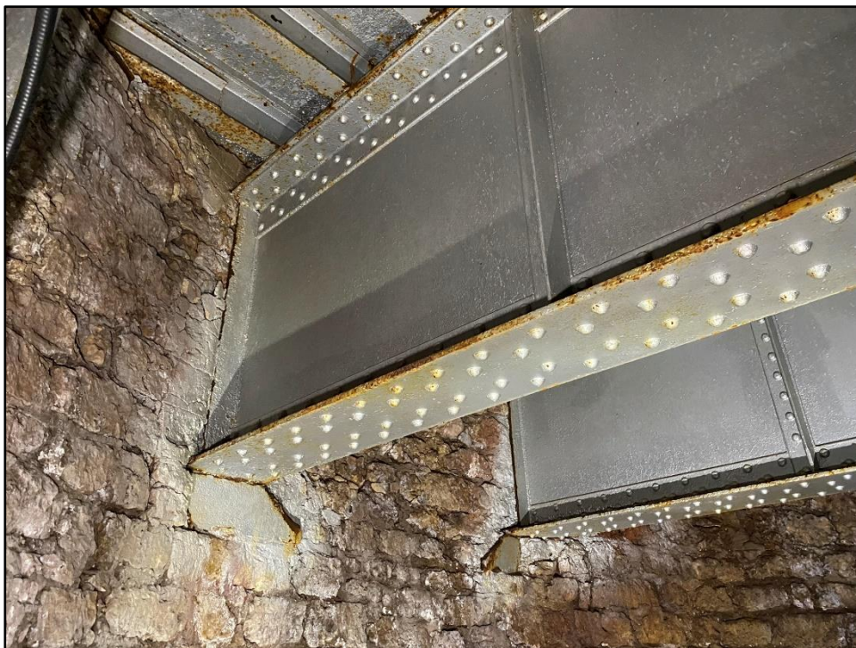
Photo 3: Steel plate girder supports
