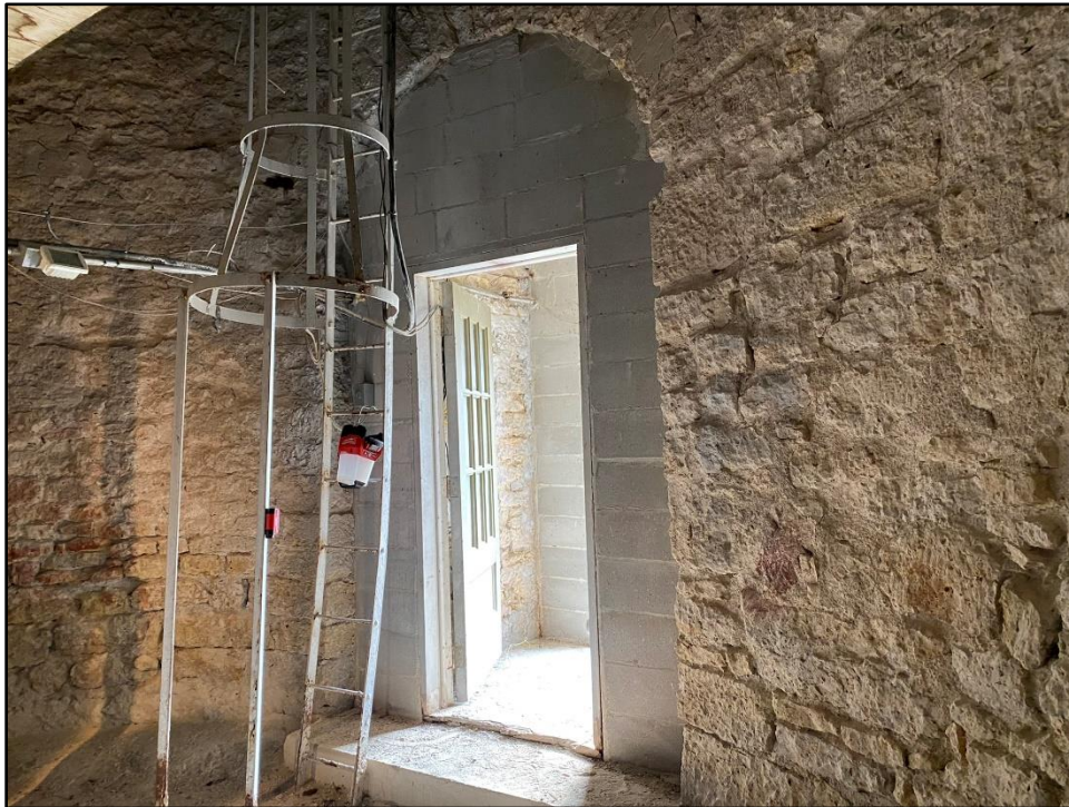
Photo 10: Modified entry door/wall
