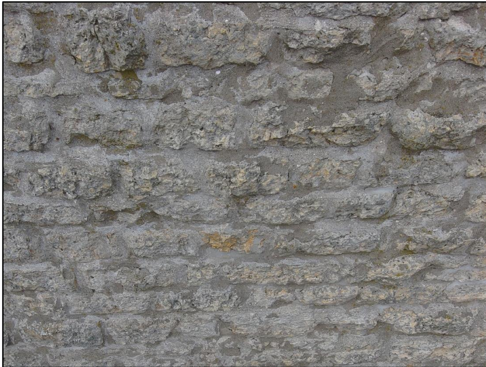
Photo 26: Repointed joints at mid-height of tower
