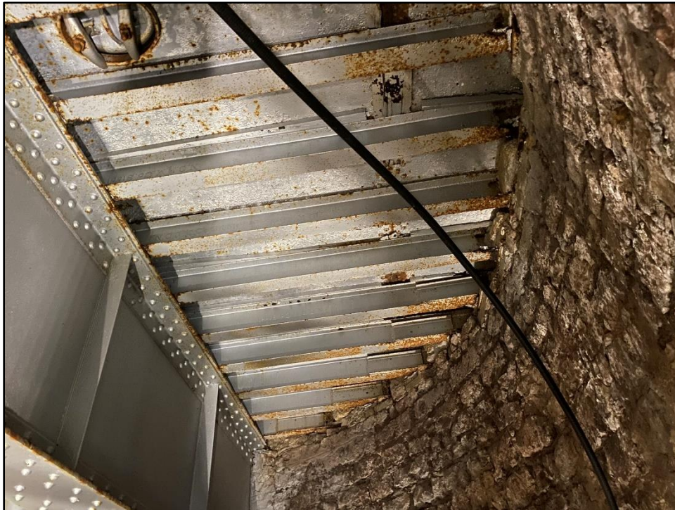
Photo 2: Steel beams below tank
