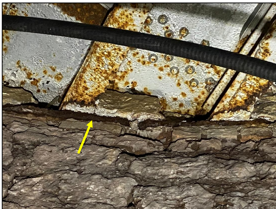
Photo 32: Close up of tank supports at wall
