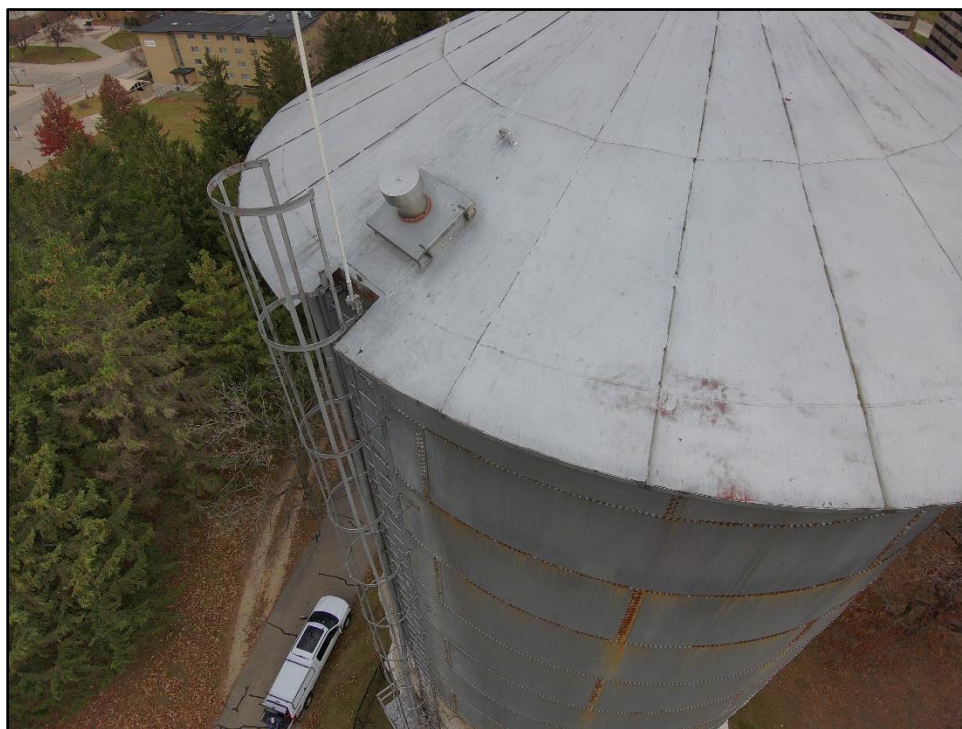
Photo 9: Exterior ladder to tank
